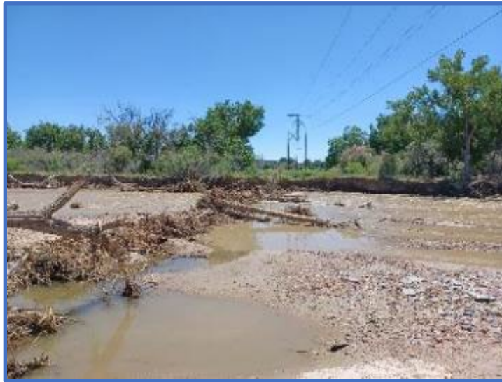
Photo 1 – Creek Conditions at Waterline Bollards
