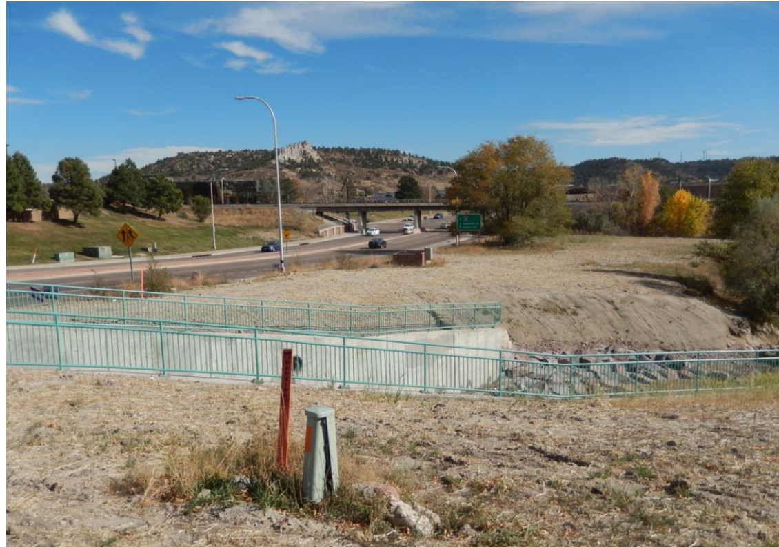
Figure 43. NRR-2: Levee Installation at South Rockrimmon Boulevard Downstream of Pro Rodeo Drive
