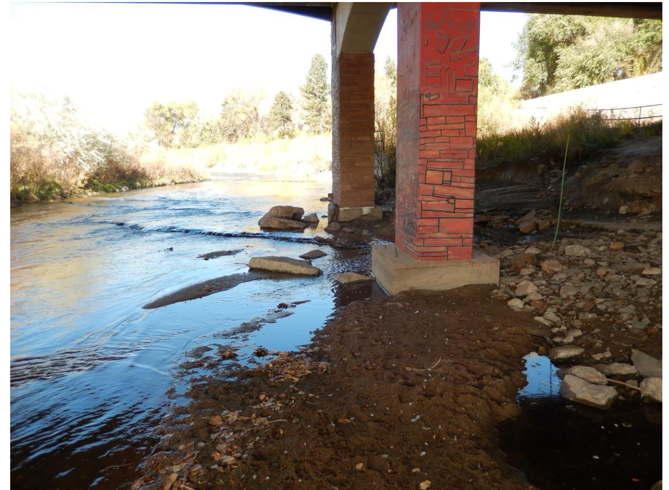
Figure 35. MCM-8: Uintah Bridge Bank Stabilization
