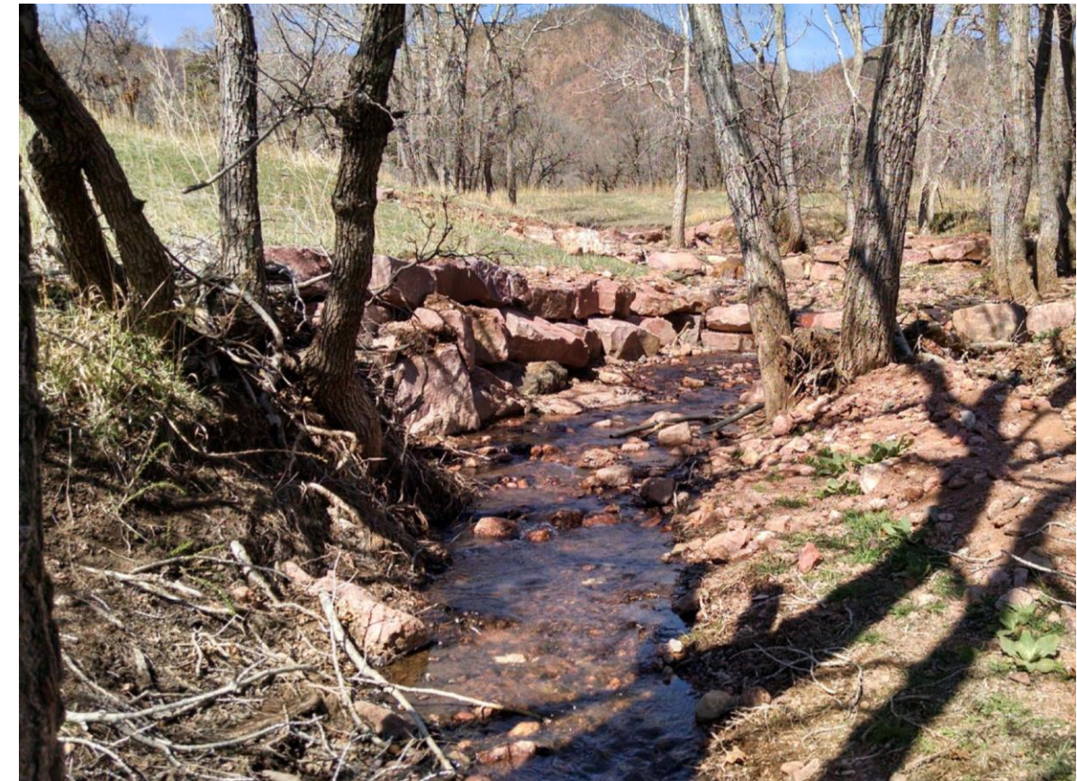
Figure 67. Constructed Rock Vane on North Douglas Creek
