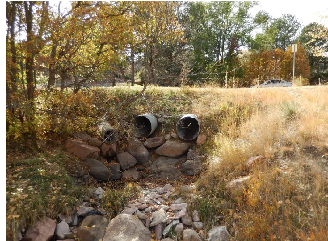
Figure 42. NRR-1: Culvert Replacement at War Eagle Lane
