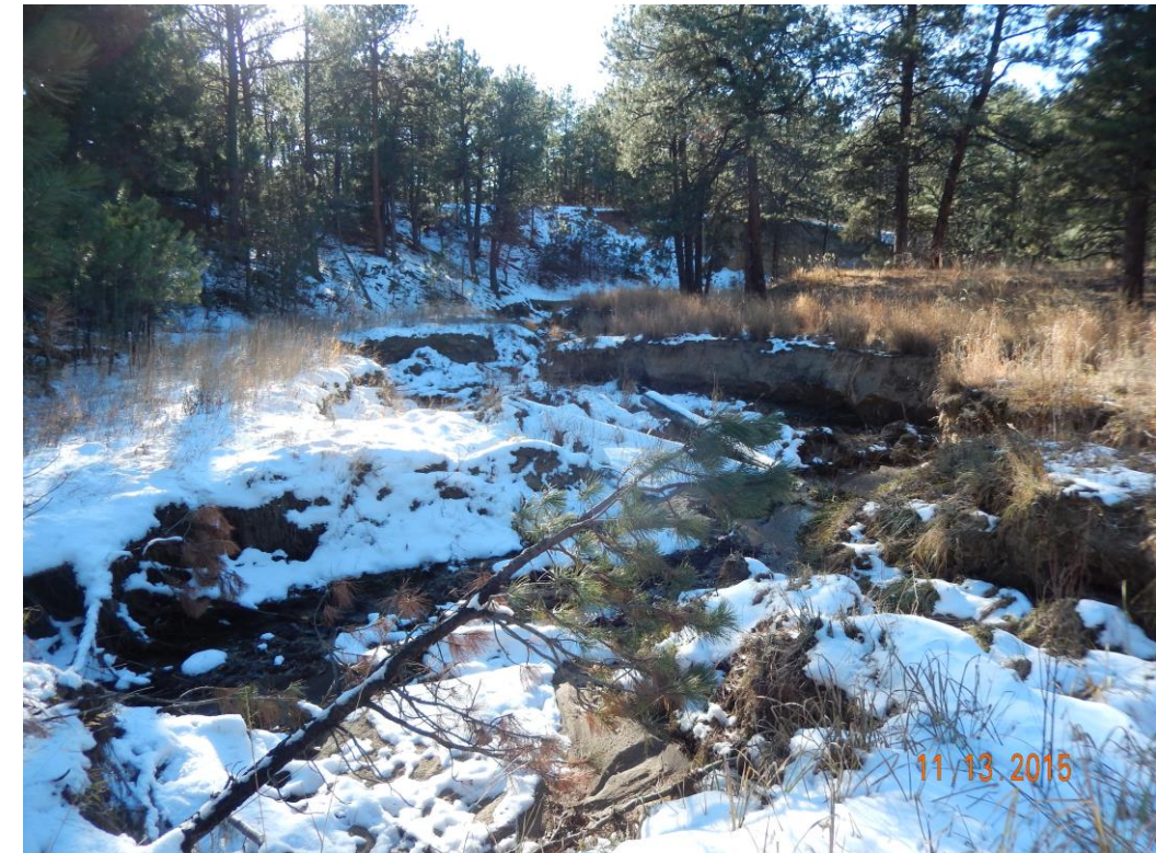
Figure 38. MT-3: Stabilize Headcutting on Middle Tributary Downstream of I-25
