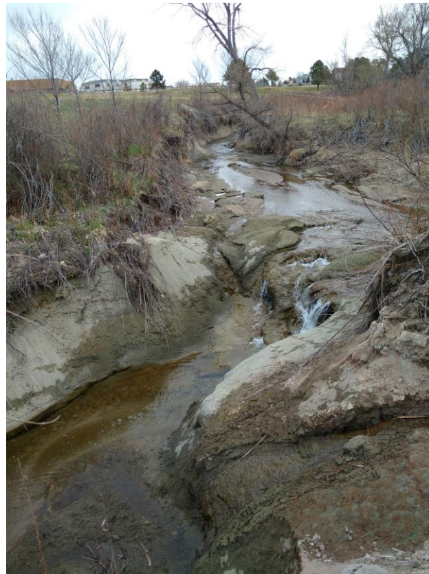
Figure 48. PC-5: Stabilize Headcutting on Pine Creek Upstream of Briargate Boulevard
