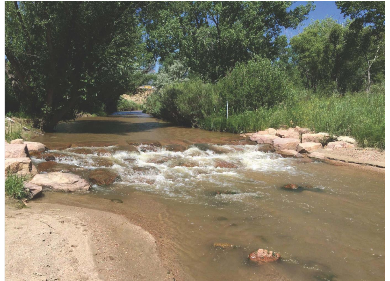
Figure 71. Constructed Boulder Drop Structure on Monument Creek
