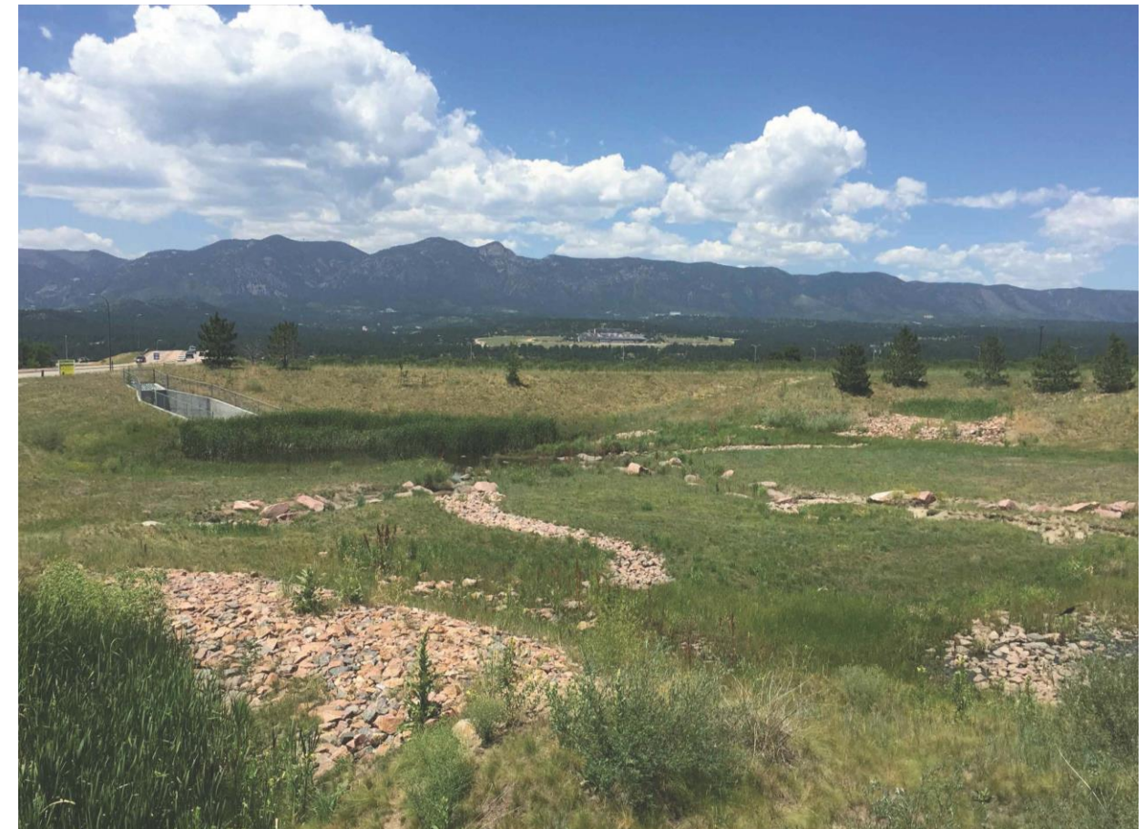
Figure 74. Existing Full spectrum Detention Facility at Interquest Parkway and I-25
