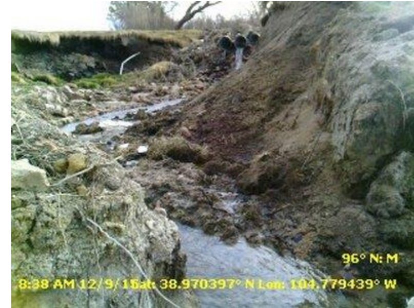
Figure 47. PC-4: Stabilize Headcutting on Pine Creek Golf Course at Trail Crossing
