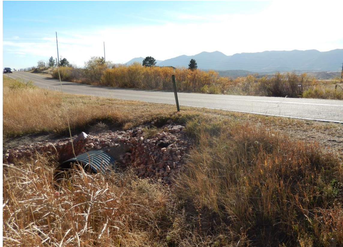
Figure 54. TC-2: Culvert Replacement at Teachout Creek and Old Denver Highway
