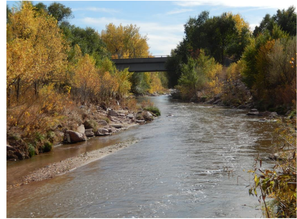
Figure 33. MCM-6: Flood Risk Reduction at West Polk Road Bridge at Monument Creek
