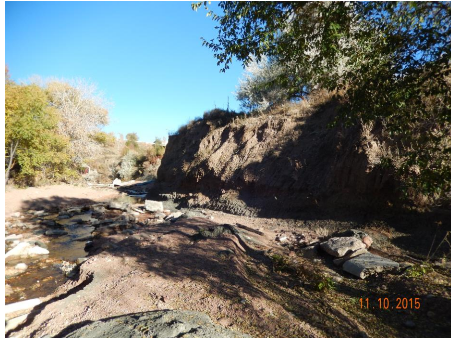
Figure 41. NDC-1: North Douglas Small Drop Structures East of I-25
