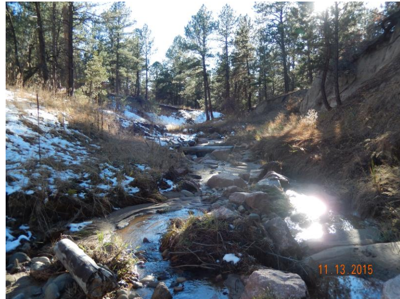
Figure 39. MT-4: Middle Tributary Small Drop Structures West of I-25
