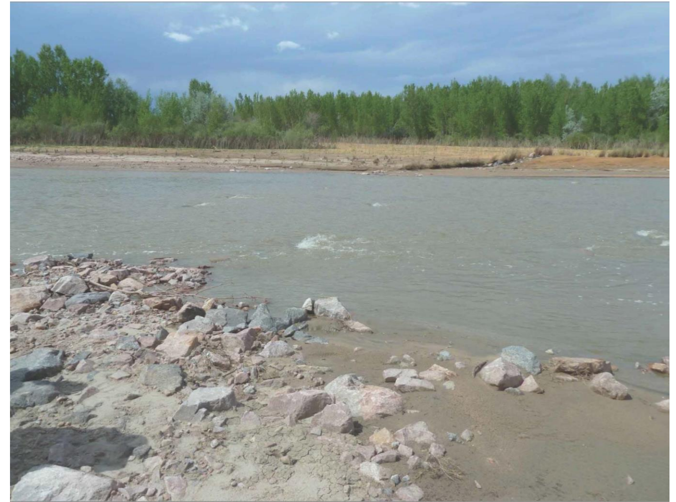
Figure 69. Constructed Riffle on Fountain Creek
