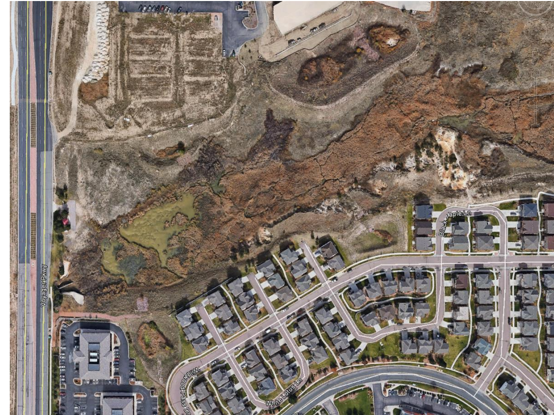
Figure 19. BS-4: Black Squirrel Detention Retrofit Upstream of Voyager Parkway
