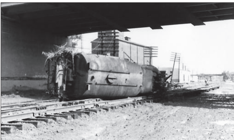
A railroad tanker rests on its side after floodwaters receded from the June 17, 1965, flood on Fountain Creek.
