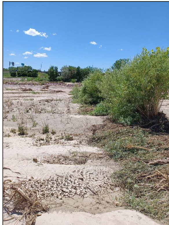
Figure 36. On-site brush layering.
