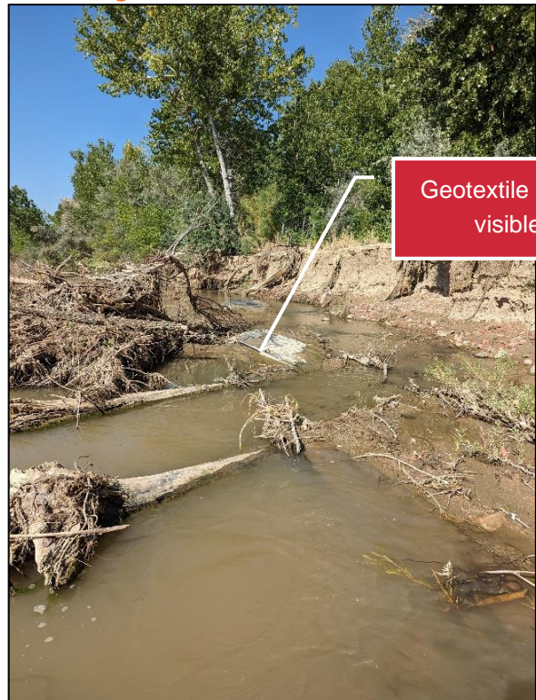
Figure 24. Soil Lifts removed.
