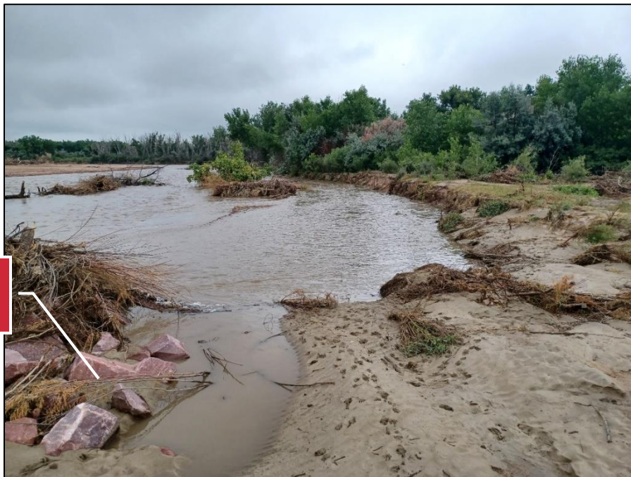
Figure 12. Upstream tie-in of riprap bank protection
