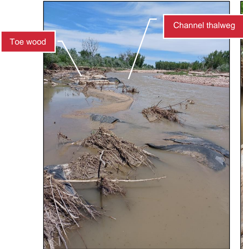
Figure 29. Remaining toewood structure.
