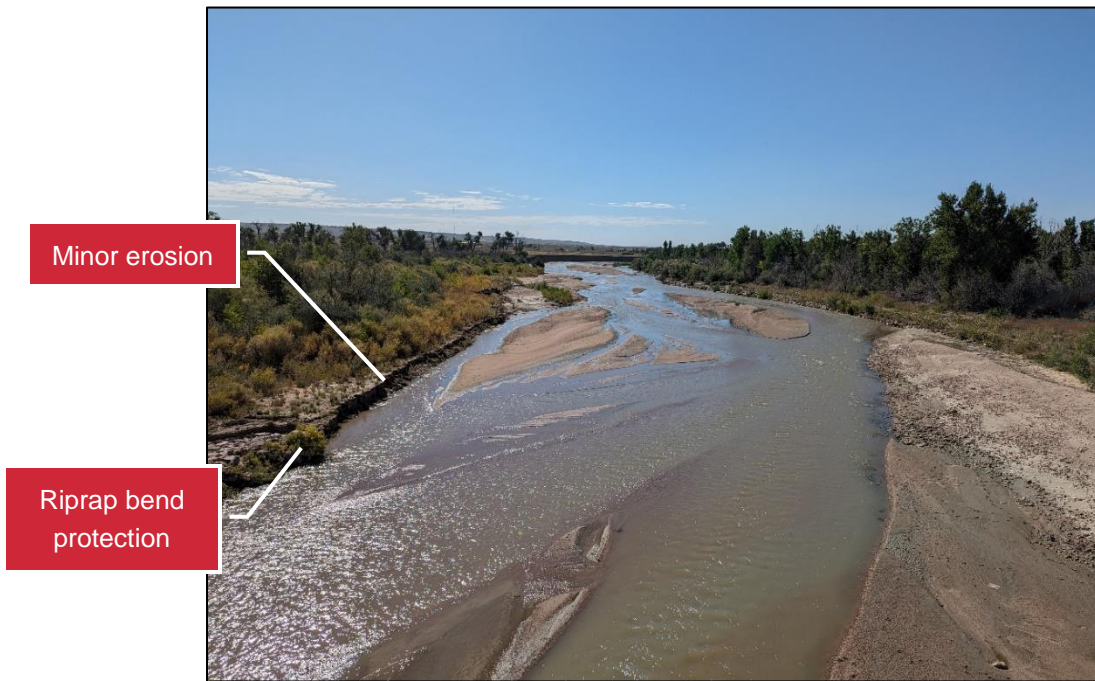
Figure 19. Eroding bank downstream of the project area.
