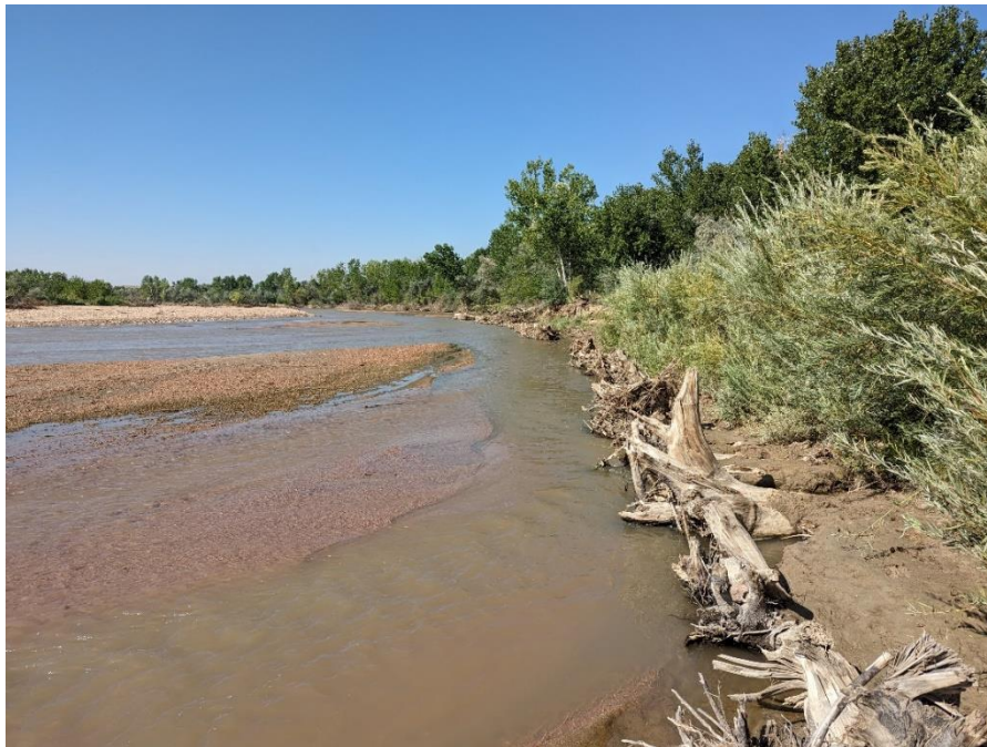
Figure 25. Intact toe wood sections.
