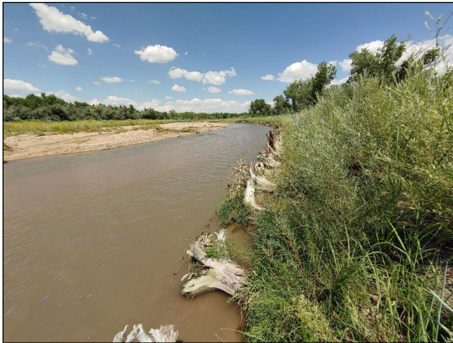
Figure 21. Bank Protection at Barr II, August 2021
