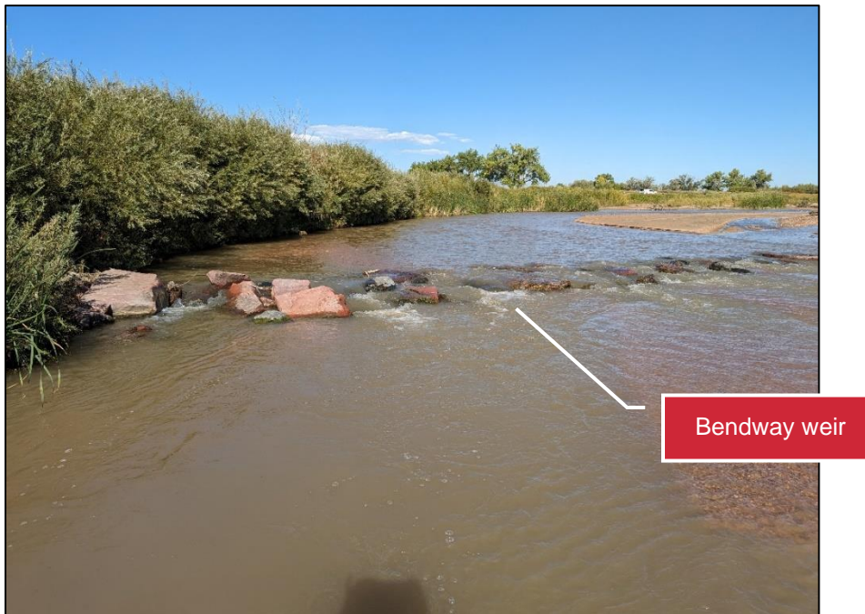
Figure 4. Buried bendway weir.
