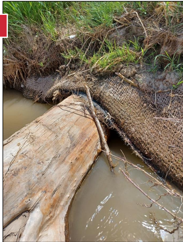
Figure 30. Soil lift over toe wood.
