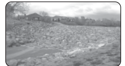
Drop Structure at Cottonwood Creek on April 28, 2004 Photo courtesy of URS.
