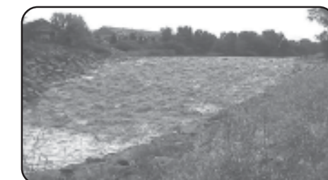
Drop Structure at Cottonwood Creek on July 16, 2004 Photo courtesy of URS.
